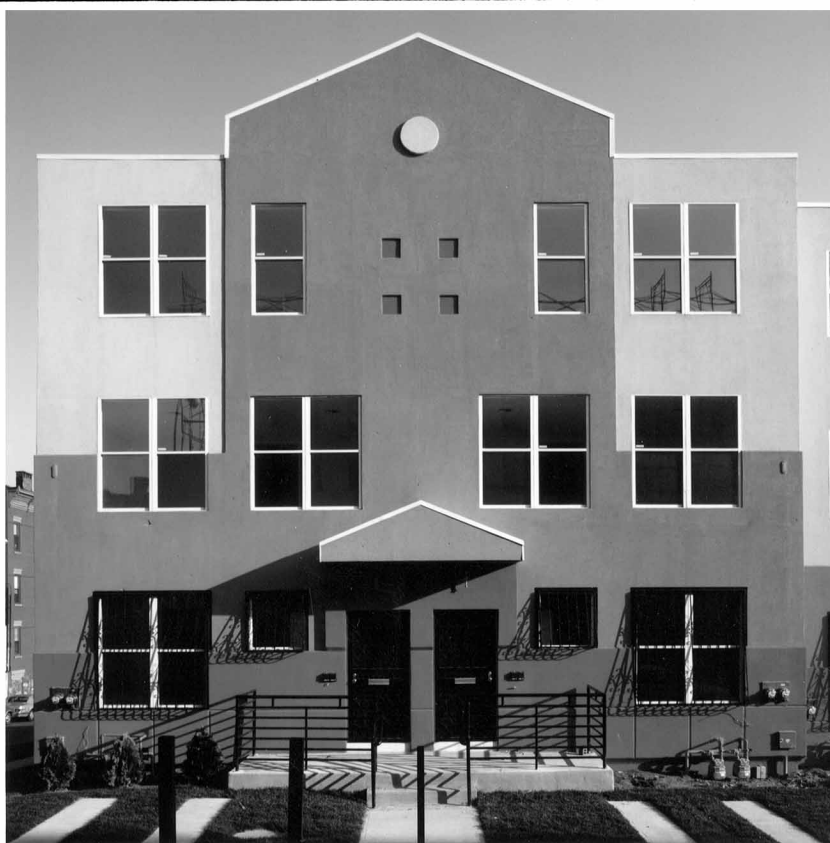
New subsidized two-family houses, done in vibrant colors, are at Melrose Avenue and East 155th Street in the Bronx.
