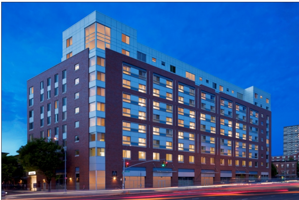
View of Atlantic Terrace from Atlantic Avenue
